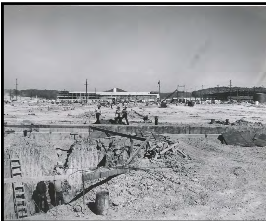
Figure 22: Foundation Construction of the X-330 Process Building, September 1953
