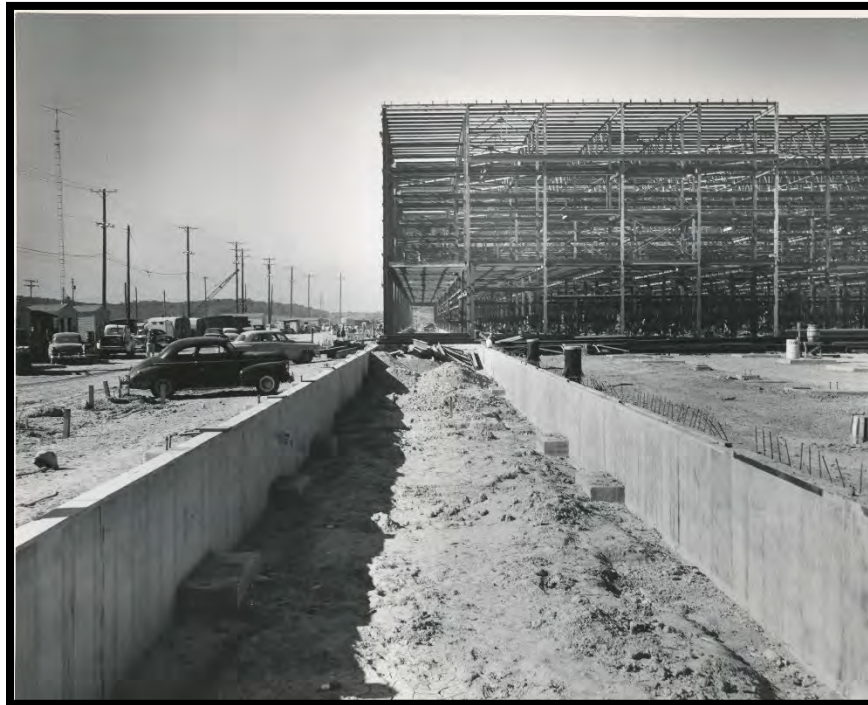
Figure 14: Foundation Construction of the X-330 Process Building, August 1953
