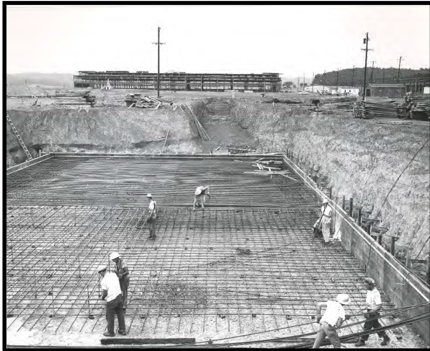
Figure 10: Foundation Construction of the X-330 Process Building, August 1953
