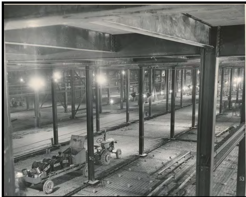
Figure 27: Cell Floor Construction of the X-330 Process Building, January 1954
