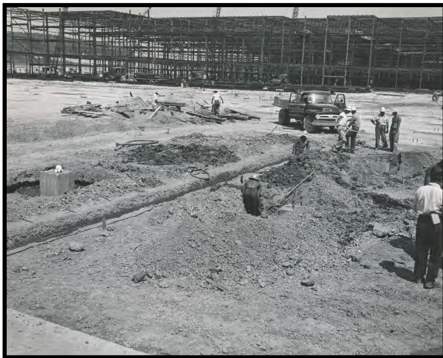
Figure 18: Foundation Construction of the X-330 Process Building, August 1953
