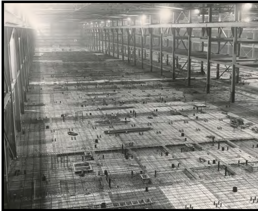
Figure 26: Cell Floor Construction of the X-330 Process Building, January 1954
