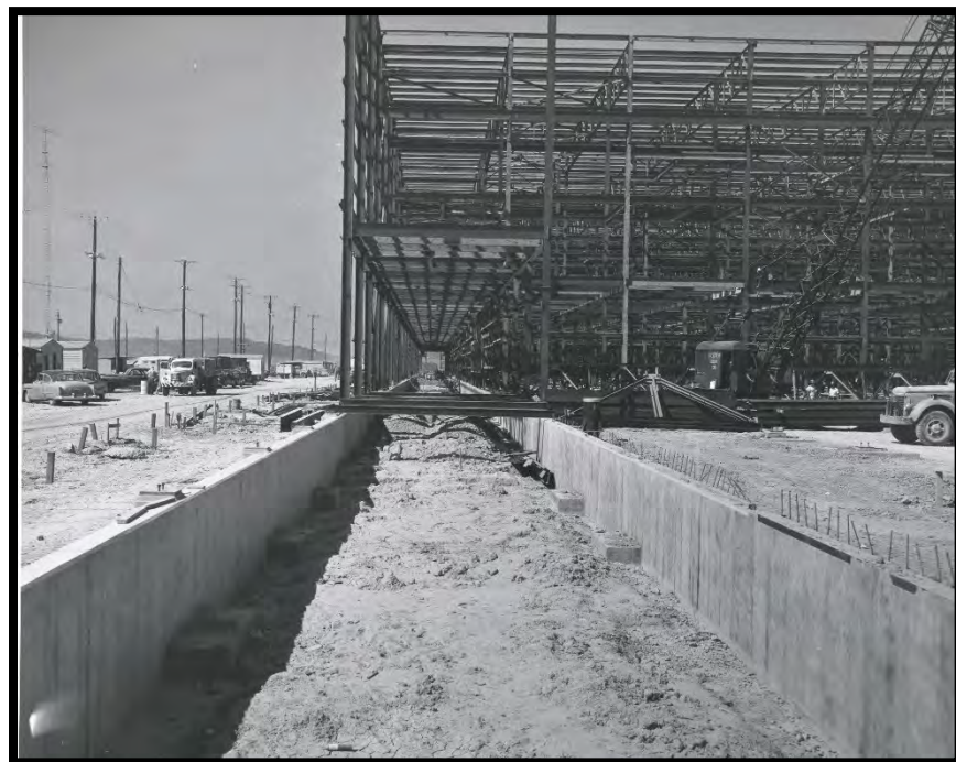
Figure 15: Foundation Construction of the X-330 Process Building, August 1953
