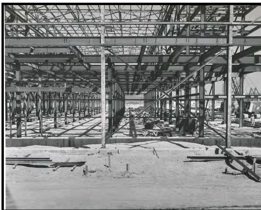
Figure 9: Steel Framework Construction of the X-330 Process Building, August 1953
